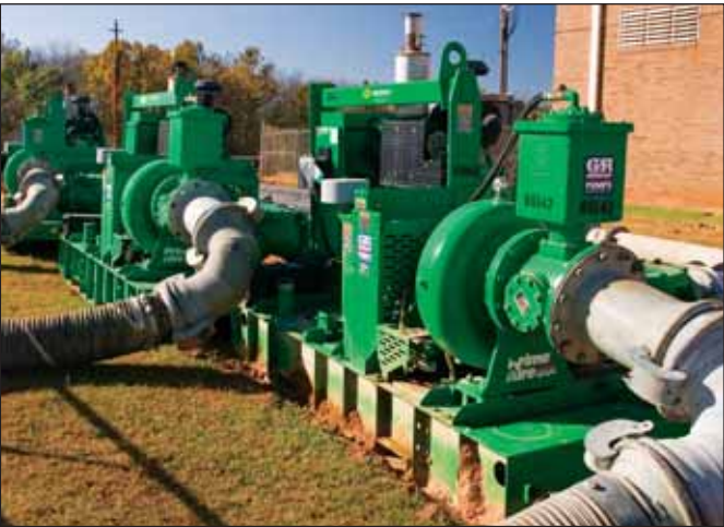
(3) Gorman-Rupp 12" x 12" Diesel Trash Pumps Working on a municipal bypass project
