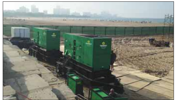
MQ Power 320 kW Industrial Generators Temporary power for a construction site
