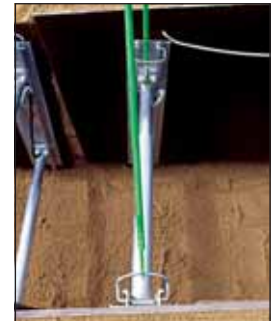
Installation and removal are performed from the top of the trench.
