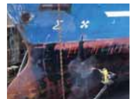
Maritime Power Plant
