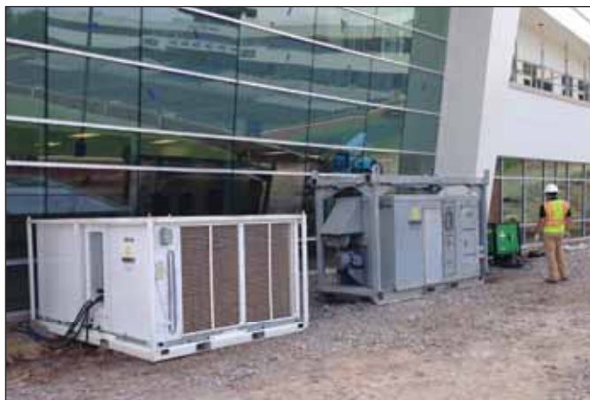
MobileCool MOB-250 25-ton Industrial Air Conditioner Temporary cooling application at a job site
