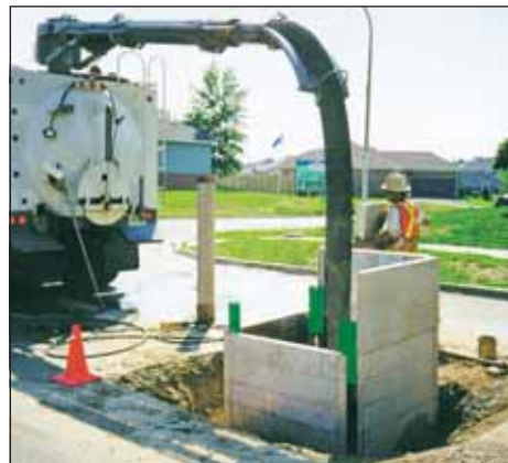
Aluminum lite shields are extremely versatile and adaptable to a wide range of applications
