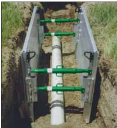
2-sided aluminum lite shield working in a pipeline application
