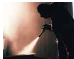
Surface Preparation Protective Coating Application
